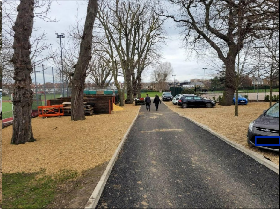
View of site from access gate
